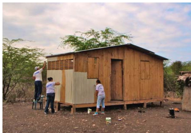
> Students and other volunteers working on construction of dwellings in Latin American slums (TECHO.ORG, 2012)
